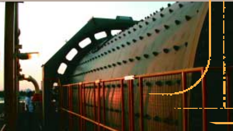
Chatree grinding mill
