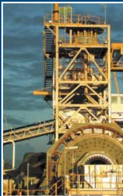
Right: Semi autogenous grinding (SAG) mill with cyclone tower behind
