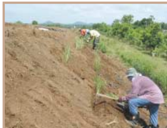
Planting vitiver grass as erosion control on bund wall
