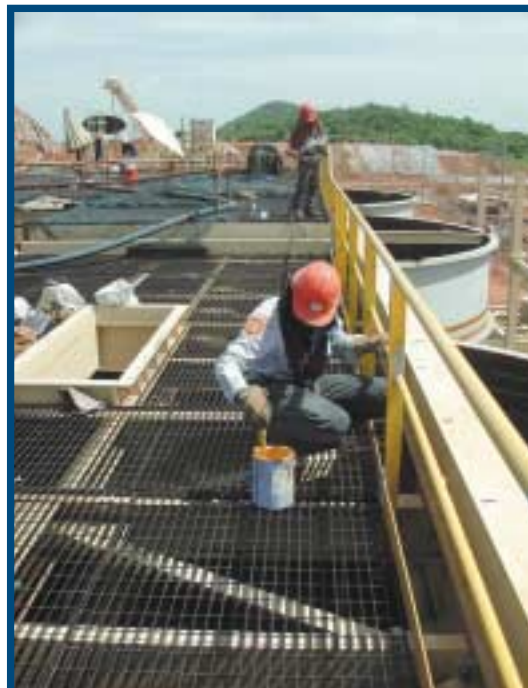
Installing safety guards above leach tanks
