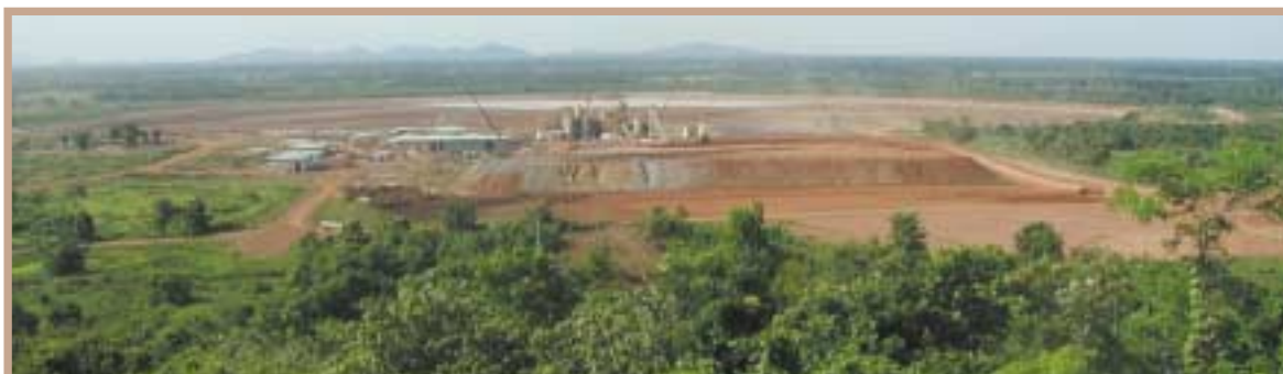
Plant site nearing completion in September 2001
