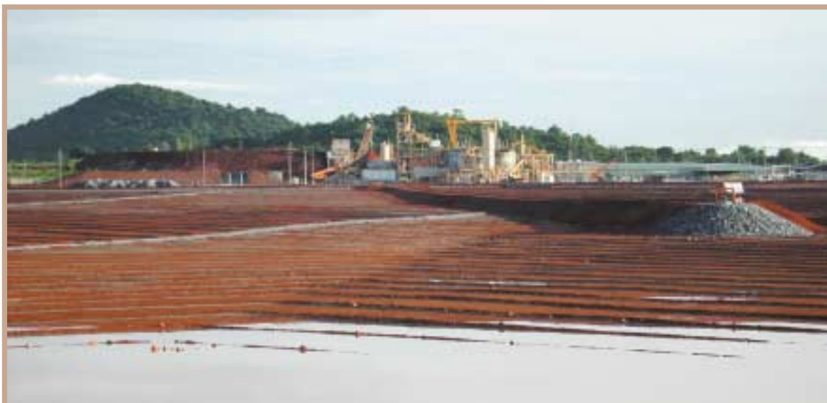
View north over project towards A Prospect hill
