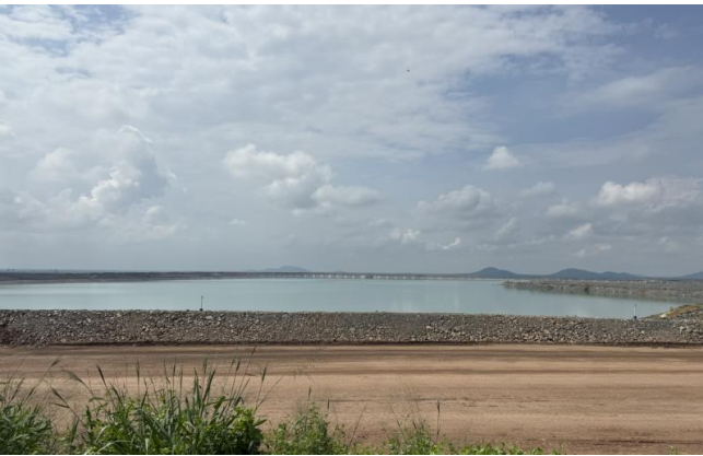
Figure 4: TSF1 – sufficient capacity for the current LOMP. Tailings storage for any mine life extension can be facilitated through purchase of additional land south of TSF2
