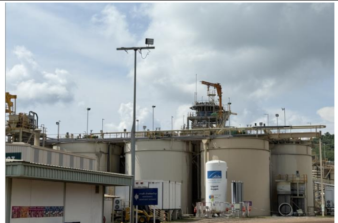
Figure 7: Plant 2 leach tanks - Plant 2 is main contributor to plant performance with rated capacity of 2.7Mtpa but currently running >3Mtpa
