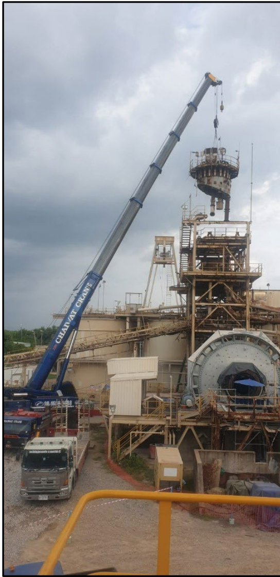
Removal of the Cyclone separator for replacement from Plant #1.
