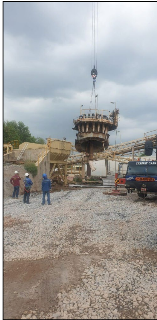
Removal of the Cyclone separator for replacement from Plant #1.
