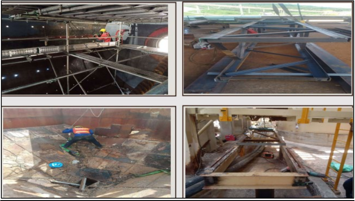
Grinding Circuit repairs above (left to right): SAG mill rubber lining removal, structure frame for conveyor CV09, repairs to conveyor hopper and conveyor frame repairs CV04.
