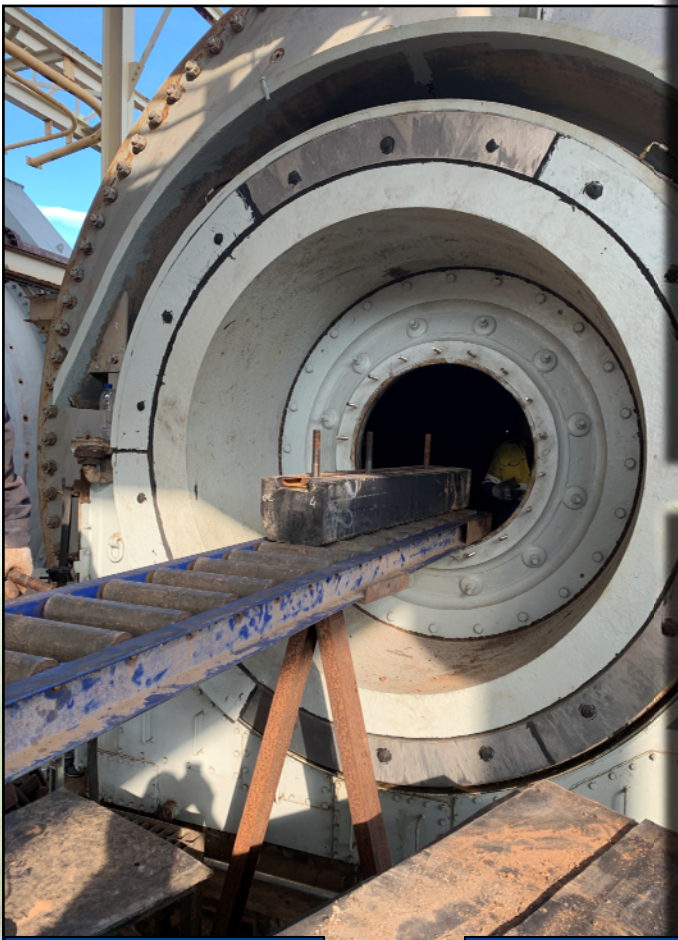
Right, from top: Ball Mill Mill reline in Progress SAG Mill
